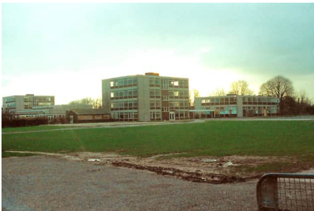
The Oak Park School Site prior to demolition
